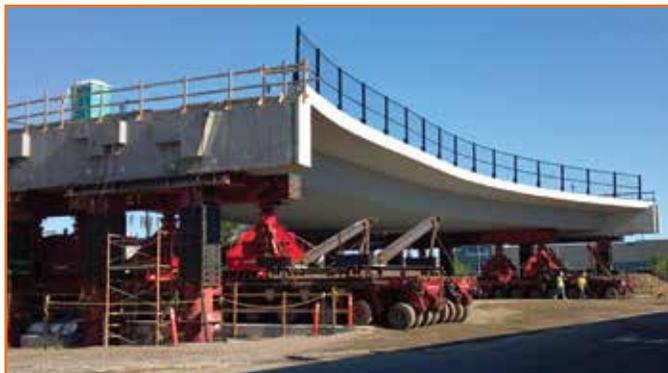
This new bridge over I-70 at Pecos was built and slid into place, reducing disruption to traffic on I-70 and saving construction costs.
