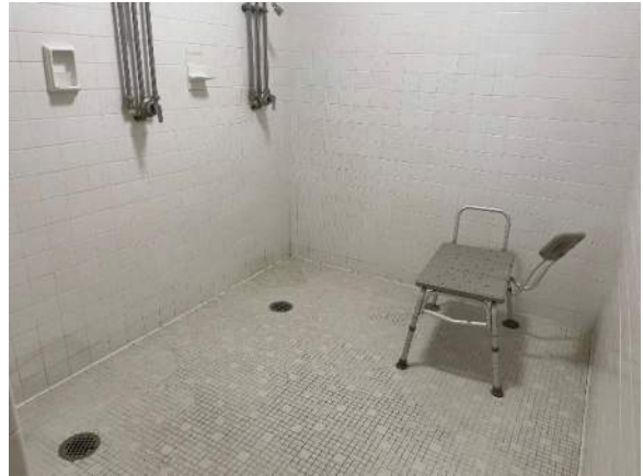
Figure 10: Typical group shower room.
