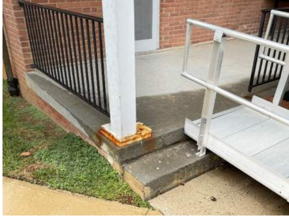
Figure 13: Temporary handicapped ramp at apartment porch.
