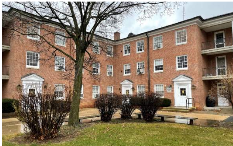
Foxwell-Moylan Hall viewed looking northwest.
