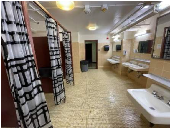
Figure 9: Second floor group toilet room.
