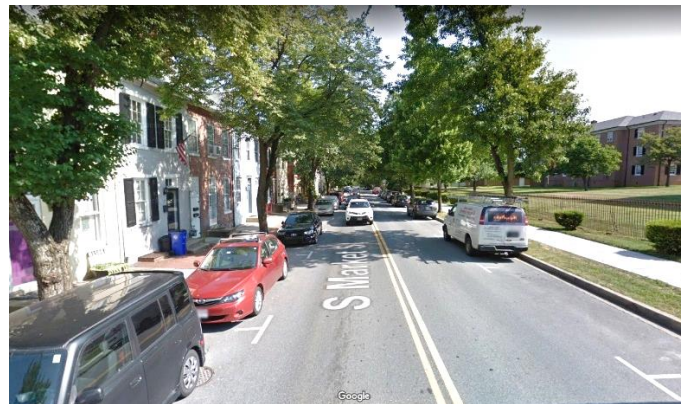
Figure 10: Site context on Market Street with existing dormitories visible at right.
