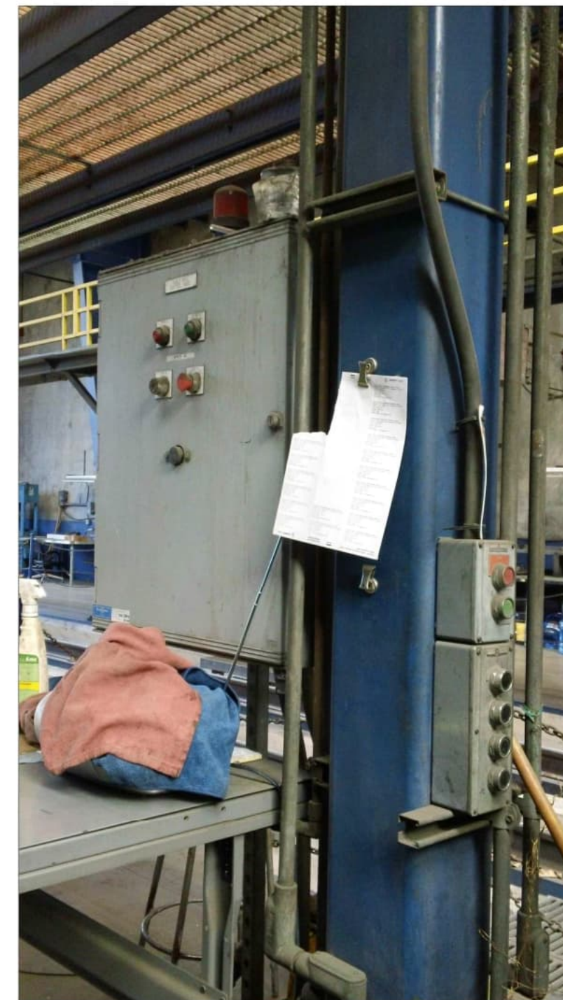
PANEL PIT 4 METRO LRT RAIL FACILITY
