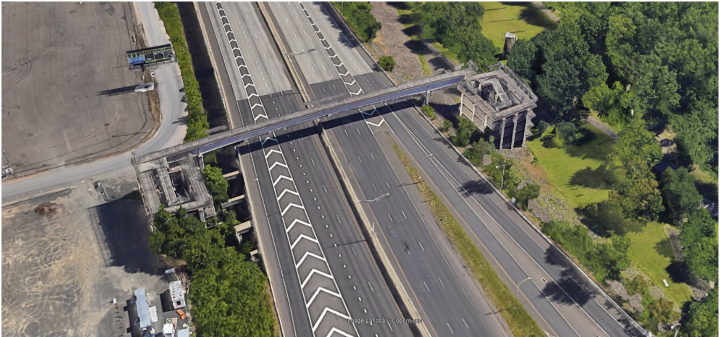
Aerial view of existing pedestrian bridge. (Image credit: Google Earth)
