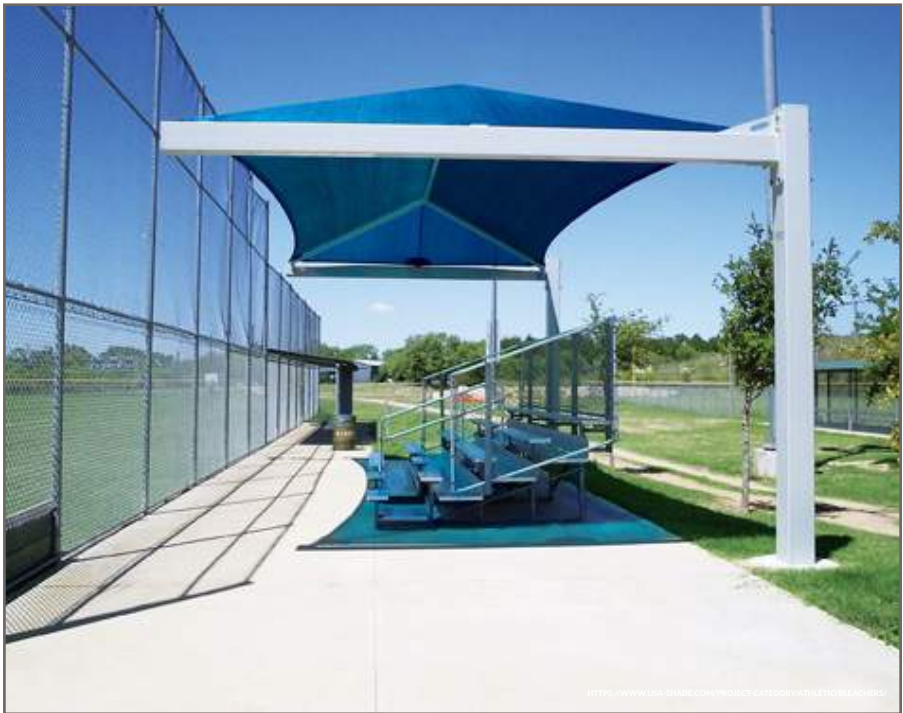
Fabric Shade Structure
