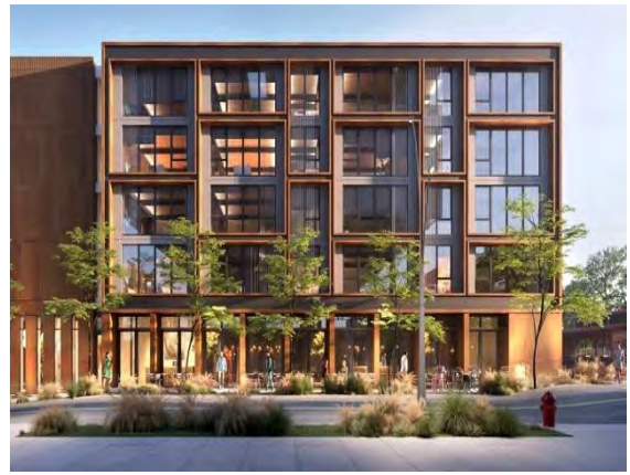
Mid-rise Residential Positioned for Condo Precedent Juno East Austin Credit: Juno / Ennead Architects
