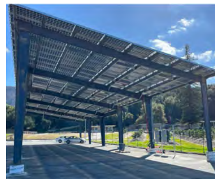
PowerShingle integrated solar and racking is specified for this system.
